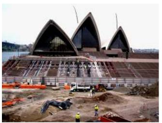
of stone that make up the steps. Once the steps were removed, they were applying a waterproof mastic material to the support structure below the steps. They were well along in this project that could be viewed from the hillside across from the Opera House, as shown on the left. The hazy sky color matched the color of the back two Opera House shells facing away from the steps and all that our camera recorded of them was the dark seam running down the ridge of each shell. A repair project
